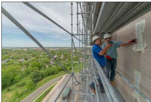
**At left, the Memorial. Above, stonemasons on the Memorial's fourth floor repair cracks in the granite. At right, new LED-based lights are installed to illuminate the Observation Deck at night.**
